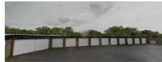
EXISTING SITE PHOTO
